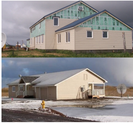
NWS Station & Residence construction on St. Paul Island
