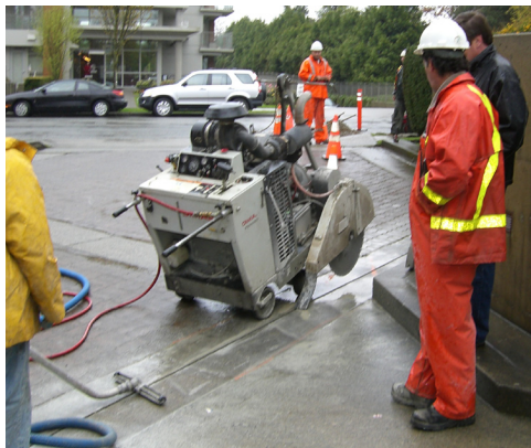
Slot cutting in roadbed for installation of MicroDuct
