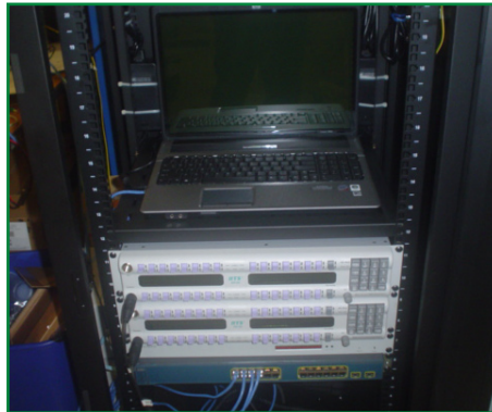
New Radio Rack ready for usage
